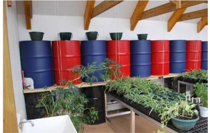
During the night or cloudy days, when the interior temperature drops, the thermal mass radiates this heat and helps maintain a suitable plant environment inside the SunCatcher. The thermal energy stored in the SunCatcher's thermal mass keeps the interior temperature well above the outdoor (ambient) temperature. This thermal mass reduces temperature fluctuations inside the SunCatcher, greatly reducing the need for daytime venting and nighttime heating.
